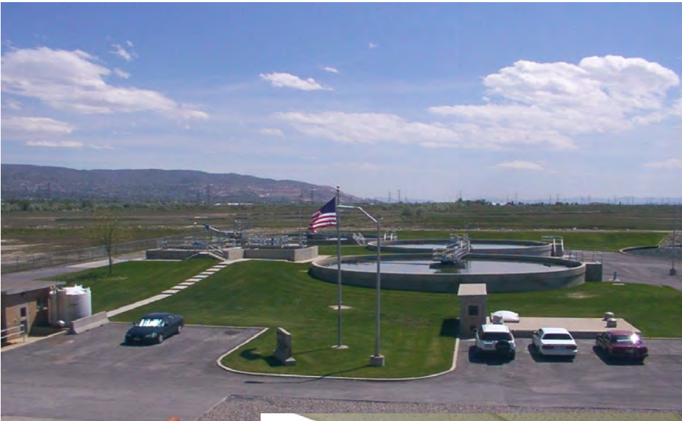
North Treatment Plant
